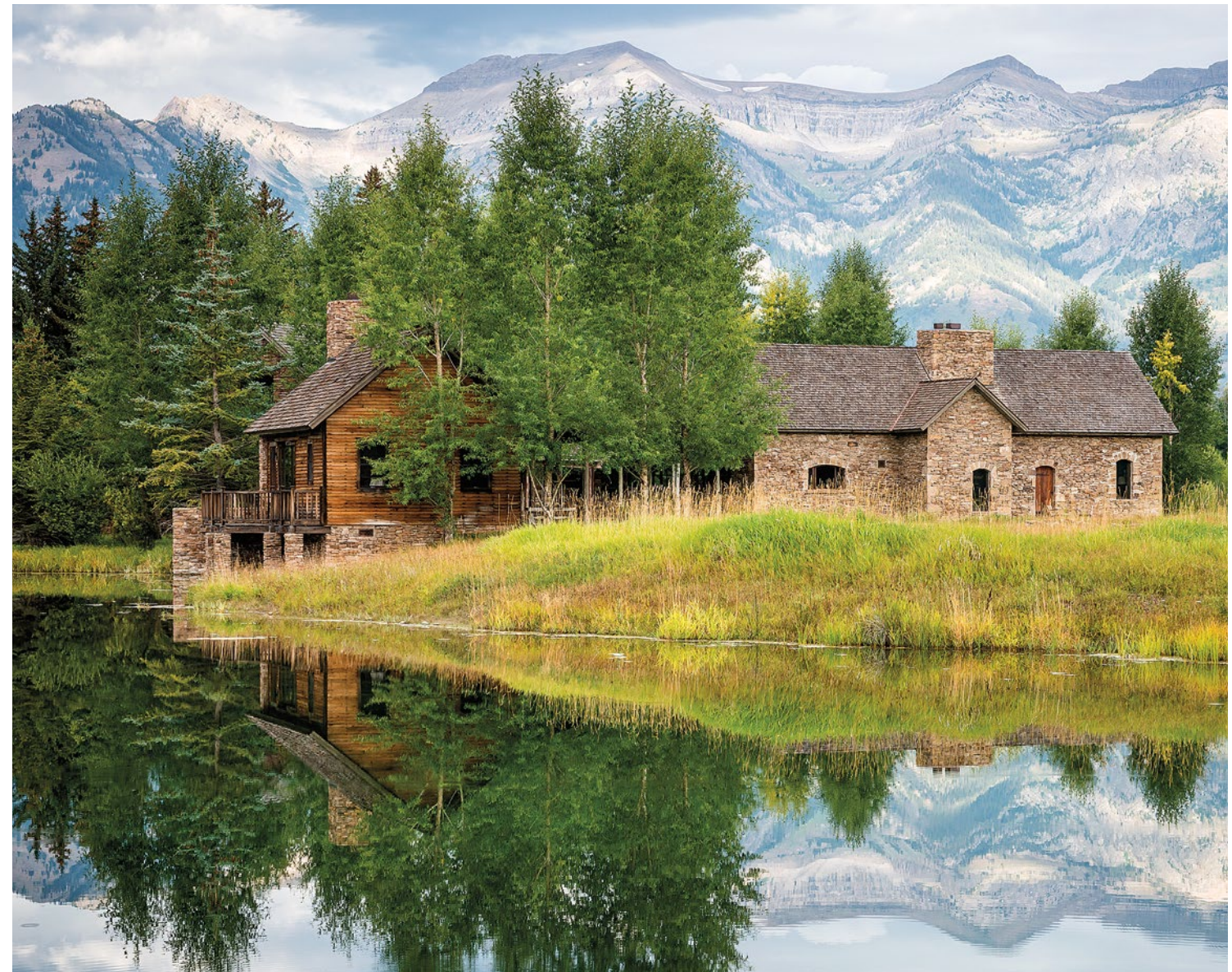
ABOVE & OPPOSITE: AN ANCIENT, NATURAL AQUIFER NOT FAR UNDERGROUND WAS CAREFULLY UTILIZED TO CREATE THE WATER FEATURES THAT GRACE THE CREAMERY. THE GLASS AND STEEL WALKWAY THAT CONNECTS THE ORIGINAL CREAMERY TO THE ADJOINING ADDITIONS UNOBTRUSIVELY BLENDS OLD WITH NEW. THE STONES USED IN THE WALKWAY FLOOR WERE RECLAIMED FROM CASTLES AND ESTATES IN YORKSHIRE, ENGLAND.
